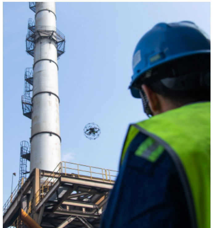
INSPECTION AT HEIGHT. The drone technology replaces manual inspection, thus eliminating complex tasks.
